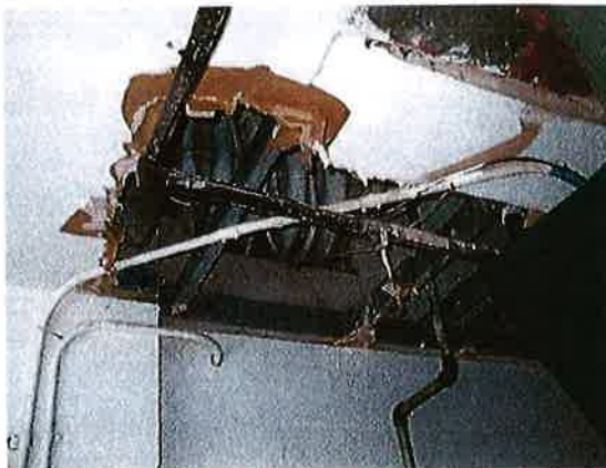
Openings in wall in trash room
